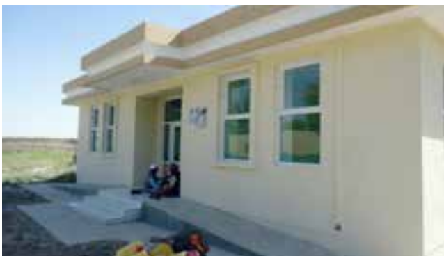
Clinic Construction, Dawlatabad district, Balkh
