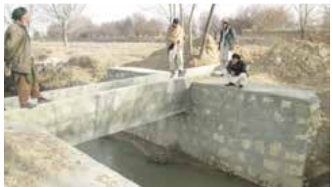
Aqueduct project, Charbolak District, Balkh
